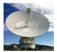
Figure 5. The 70-meter (230 feet) antenna at the Goldstone Deep Space Communications Complex in the Mojave Desert, California. This is one of many radio antennae at Goldstone, which is one of the three facilities that make up NASA's Deep Space Network. (Image courtesy: NASA/JPL)
