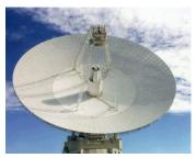
Figure 4. The 70-meter (230 feet) antenna at the Goldstone Deep Space Communications Complex in the Mojave Desert, California. This is one of many radio antennae at Goldstone, which is one of the three facilities that make up NASA's Deep Space Network. (Image courtesy: NASA/JPL)
