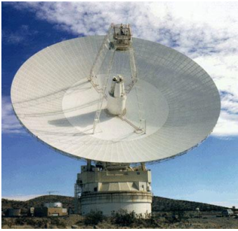
Figure 3. The 70-meter (230 feet) antenna at the Goldstone Deep Space Communications Complex in the Mojave Desert, California. This is one of many radio antennae at Goldstone, which is one of the three facilities that make up NASA's Deep Space Network. (Image courtesy: NASA/JPL)
